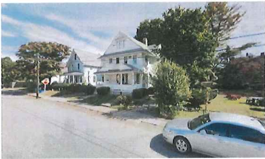
47 Oneco St Building
